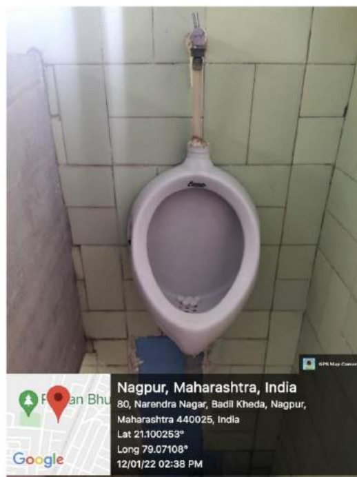
Cocks to be replaced by push buttons
